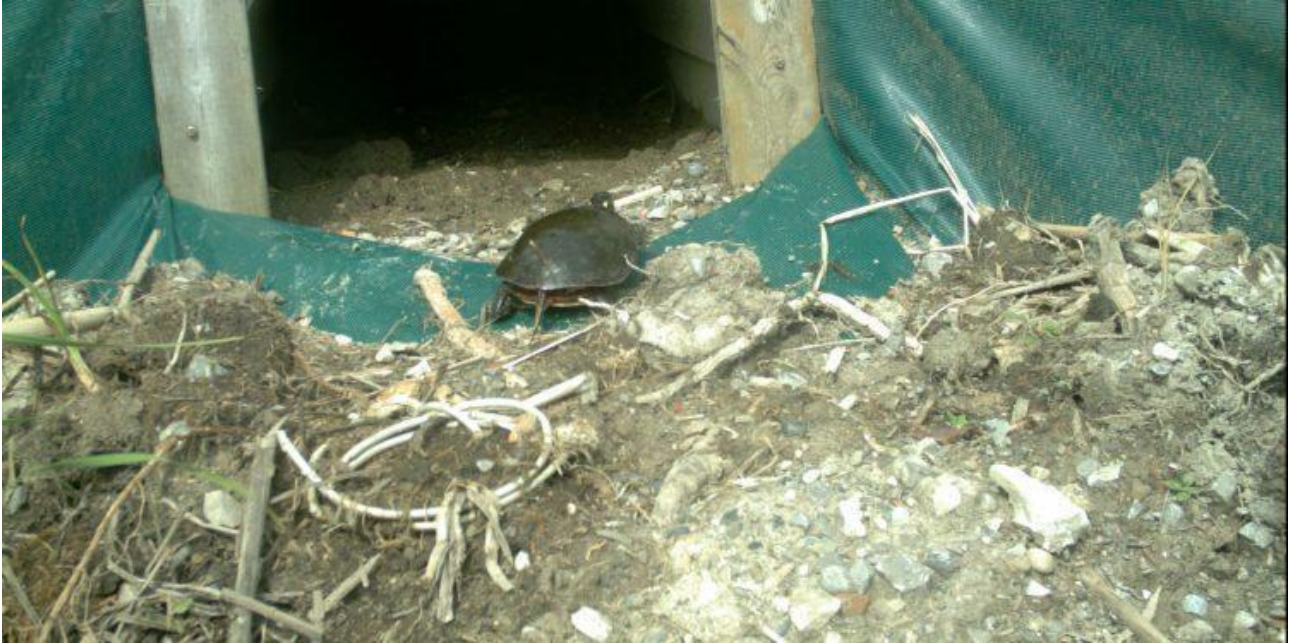
Figure 10.3 A Midland Painted turtle enters one of the new culverts that were installed under the Causeway in the fall of 2014 to enable wildlife to pass safely under the busy road 30
