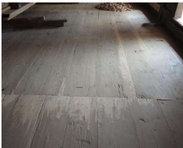
Figure 50: Timber flooring using repaired floor boards
