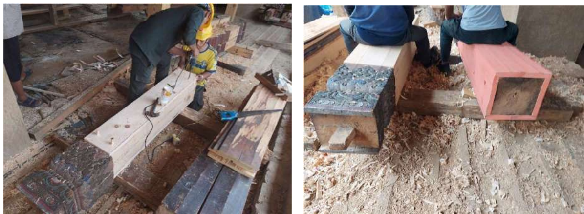
Figure 43: Repair and replacing the deteriorated part of Kachen
