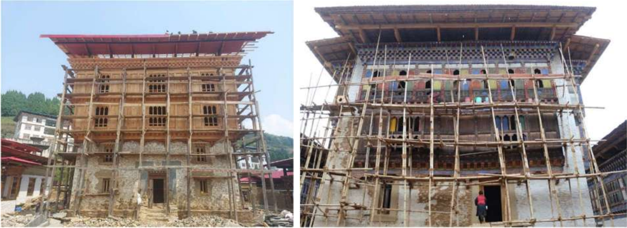
Figure 17: Timber scaffolding (Right) and Bamboo scaffolding (Left)
