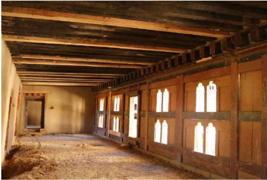
Figure 34: The unpainted Chams were reinstalled
