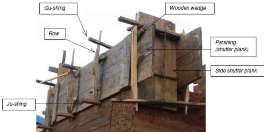
Figure 29: (a) Installation of Padom, (b) Pouring of moist soil, (c) Compaction and (d) Finished rammed earth block
