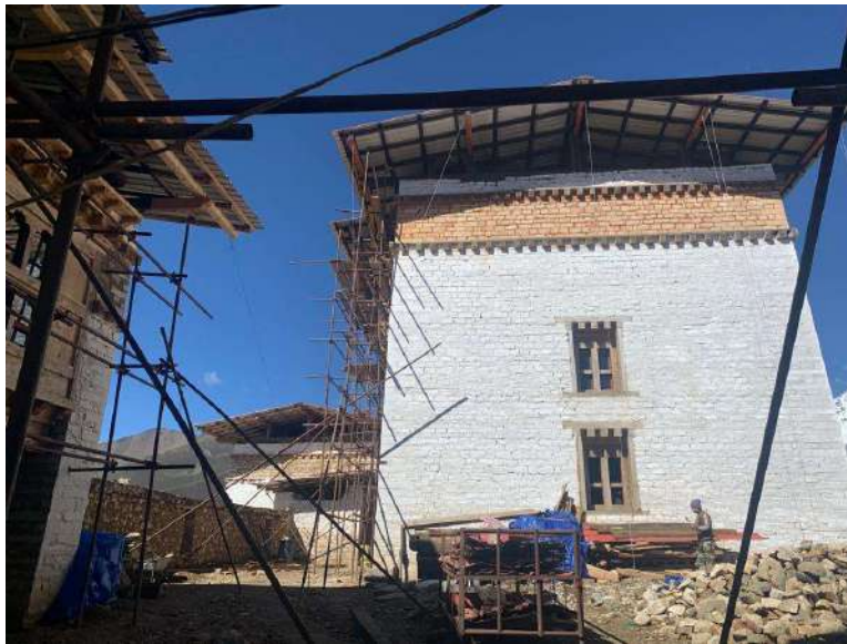
Figure 19: Steel scaffolding used in conservation project
