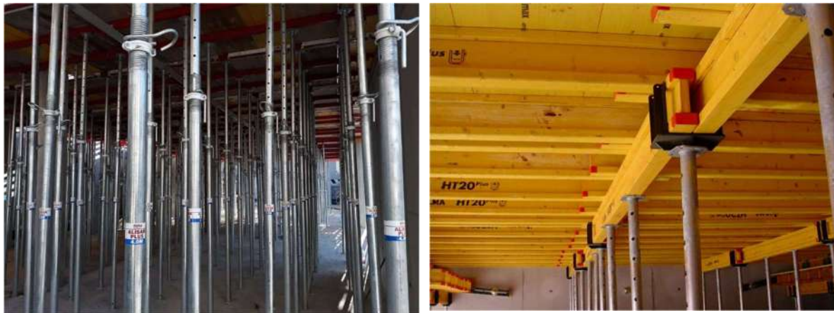
Figure 22: Steel propping
