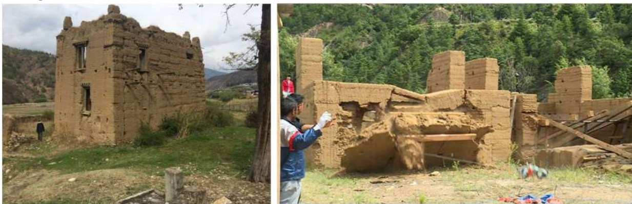
Figure 1: Demolishing of Rammed earth wall
