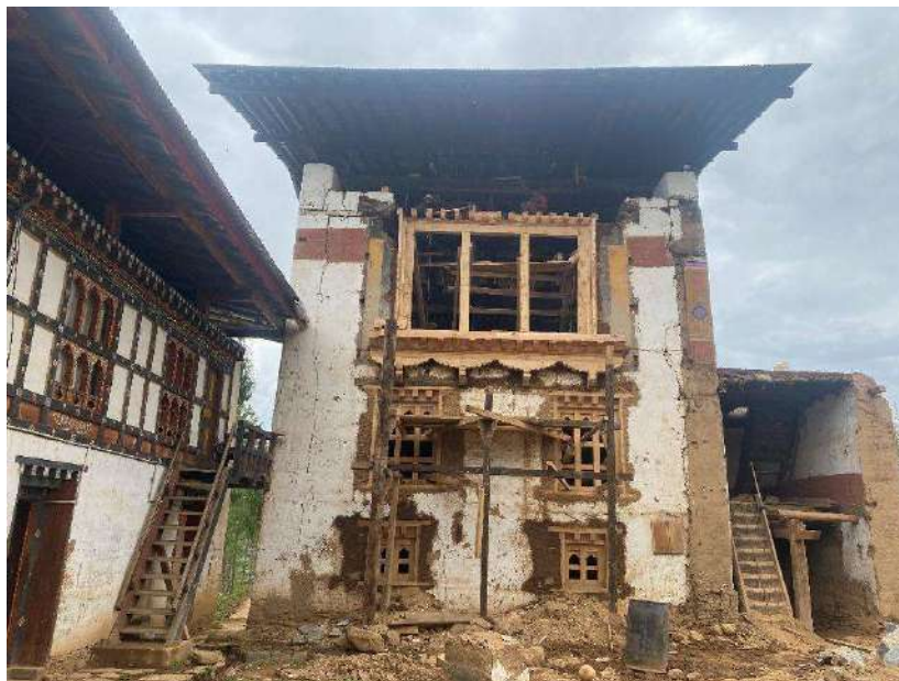
Figure 37: Reinstalled timber windows on existing wall
