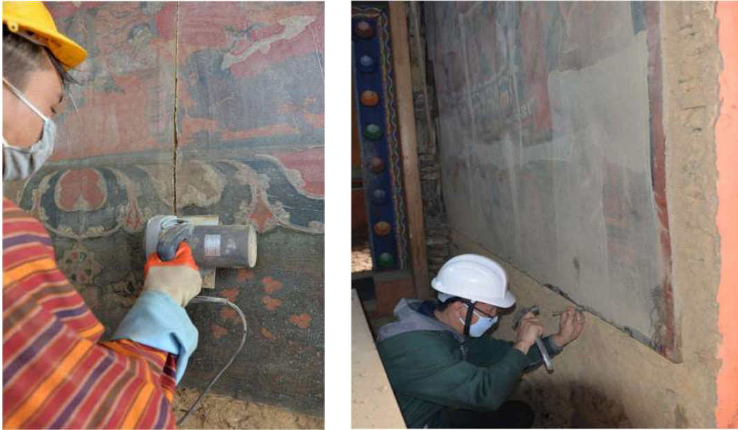
Figure 6: Clearing of the edges of murals on the stone wall
