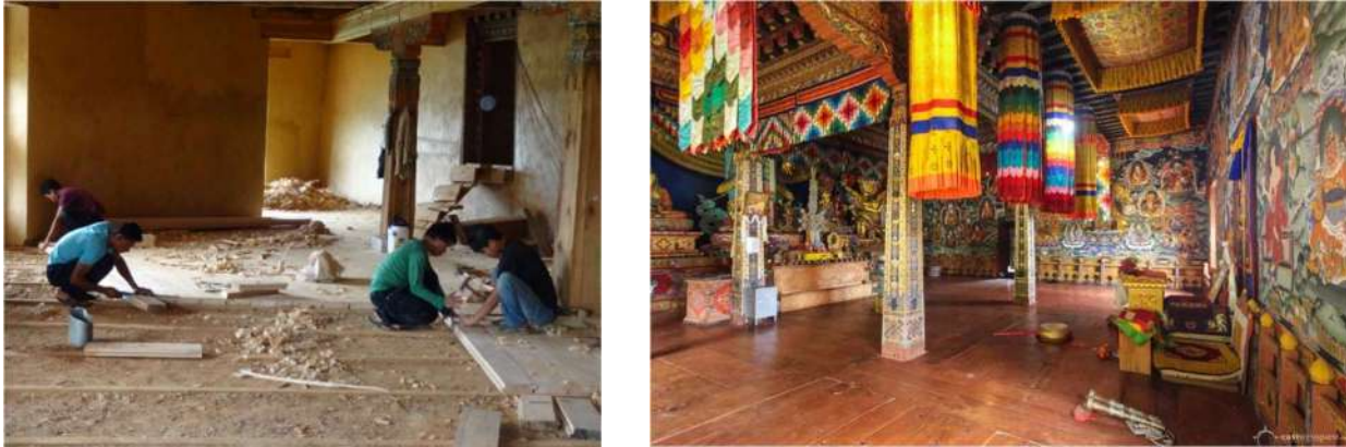
Figure 49: Laying of Thinzhi enta (left) and finished Thinzhi enta (right)
