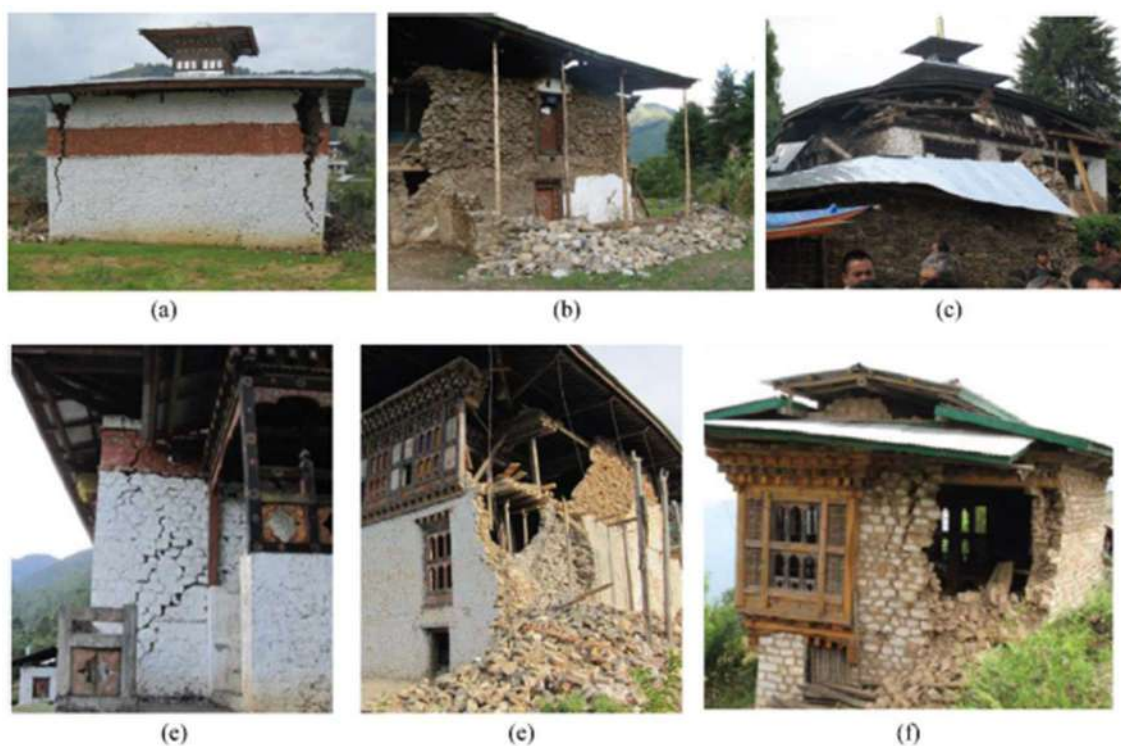
Figure 27: Common failure mechanism of stone masonry structures
