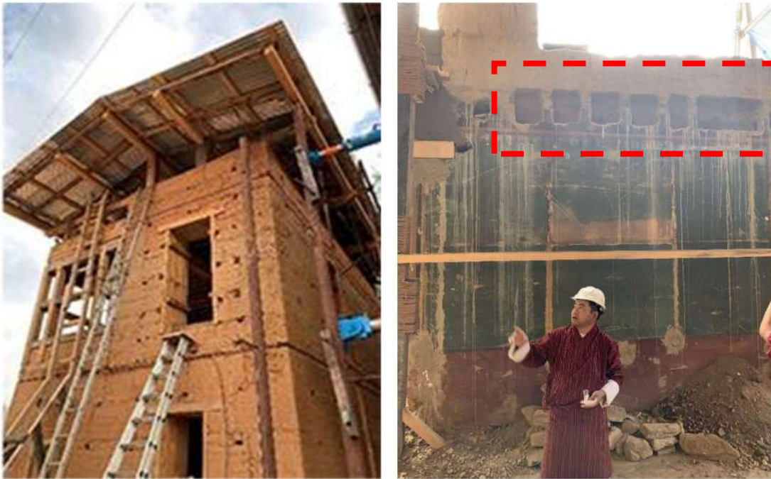
Figure 2: Cutting, trimming, shaping and leveling of rammed earth wall
