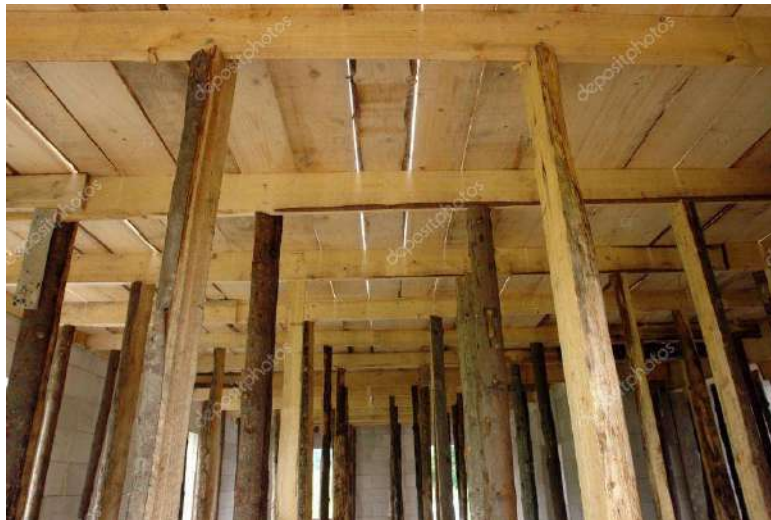
Figure 21: Timber propping
