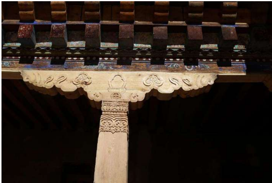
Figure 40: Replaced Kachen, Zhu and Phue with other intact timber components
