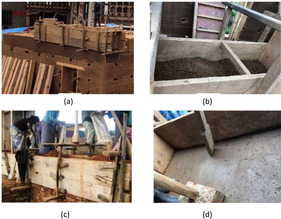
Figure 29: (a) Installation of Padom, (b) Pouring of moist soil, (c) Compaction and (d) Finished rammed earth block
