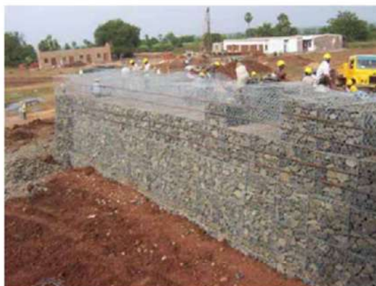
Figure 8 Lid closing procedure at site
