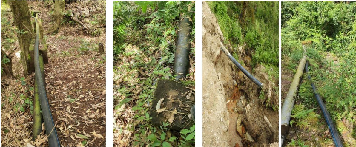
Photo 13 a-c. Existing water pipelines along the highway, overland or underground
