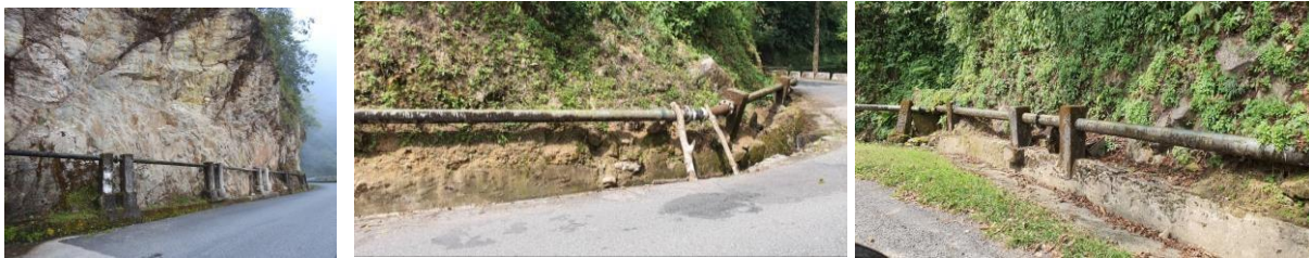
Photo 13 a-c. Existing water pipelines along the highway, overland or underground
