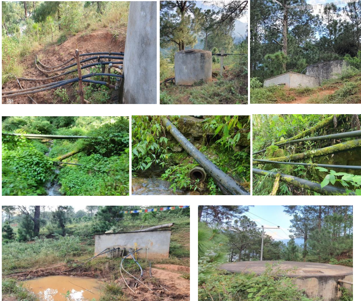
Photo 9 a – g. Existing Water Storage Tanks and Pipelines
