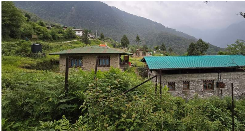
1 of 3 Sintex Tanks at the Hospital
