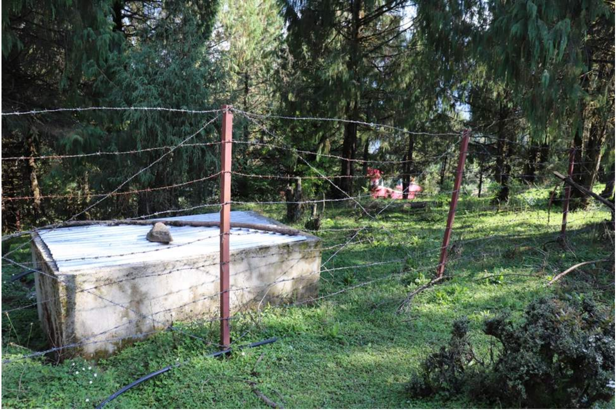
RCC Reservoir with Fencing above Gasa Dzong
