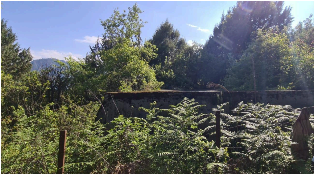
Existing water reservoir
