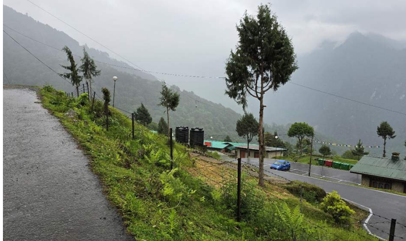
2 of 3 Sintex Tanks at the Hospital
