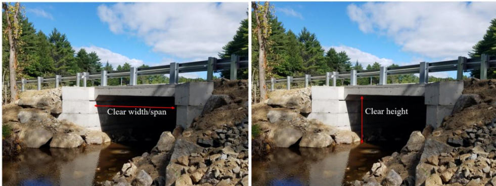
Figure 14: Consideration of structure/cross drainage opening
