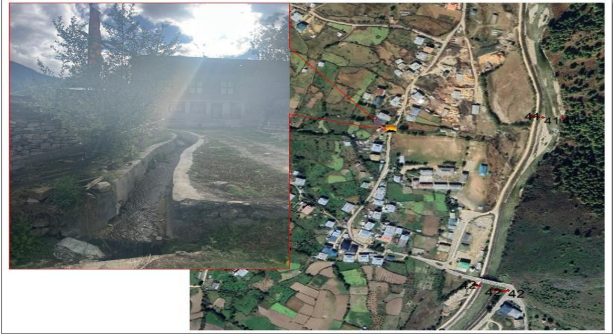
Figure 51: ingoo RCC drains
