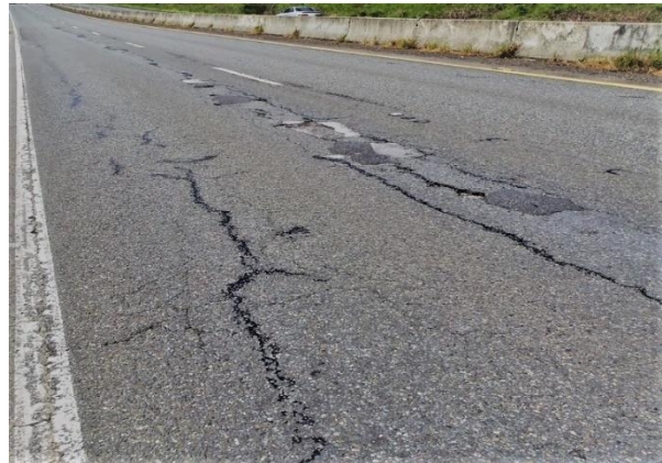
Figure 44: Meandering and Diagonal cracking on road surface
