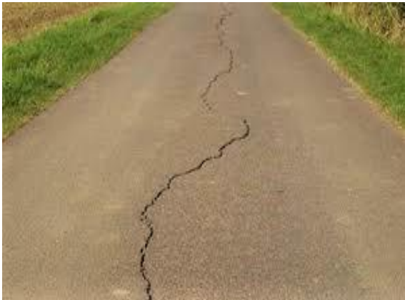
Figure 44: Meandering and Diagonal cracking on road surface
