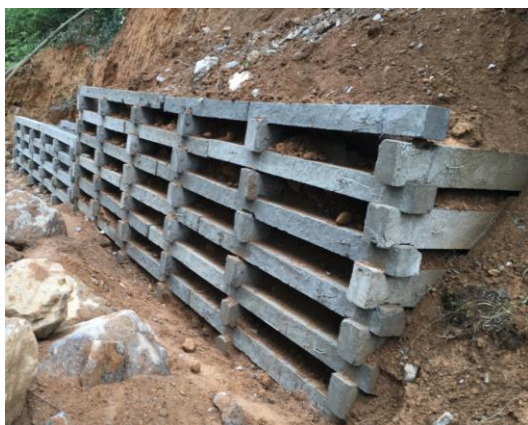
Concrete Crib Wall
