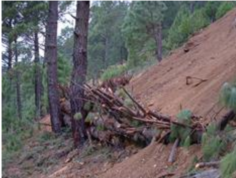
Figure 21: Timber Log barriers to catch falling materials
