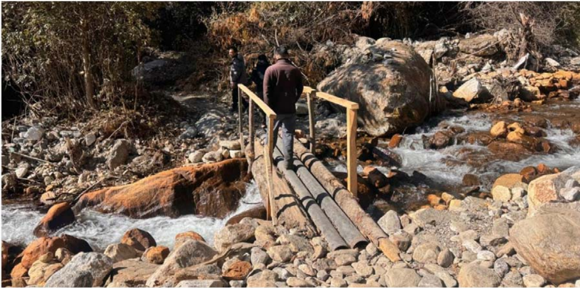
FIGURE 17: SAFETY RAILING OVER THE STREAM CROSSING TOWARDS CW-01 INTAKE SITE & CLEANED DISTRIBUTION CHAMBER AREA
