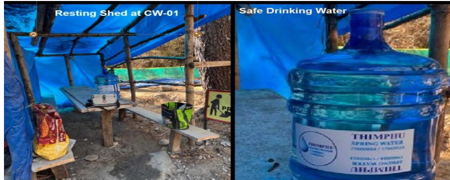
FIGURE 6: RESTING SHED PROVIDED AT THE INTAKE CONSTRUCTION SITE OF CW-01 PACKAGE
