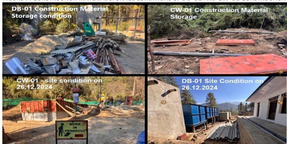
FIGURE 7: CONSTRUCTION MATERIAL STORAGE CONDITIONS OF DB-01 AND CW-01 CONSTRUCTION SITES
