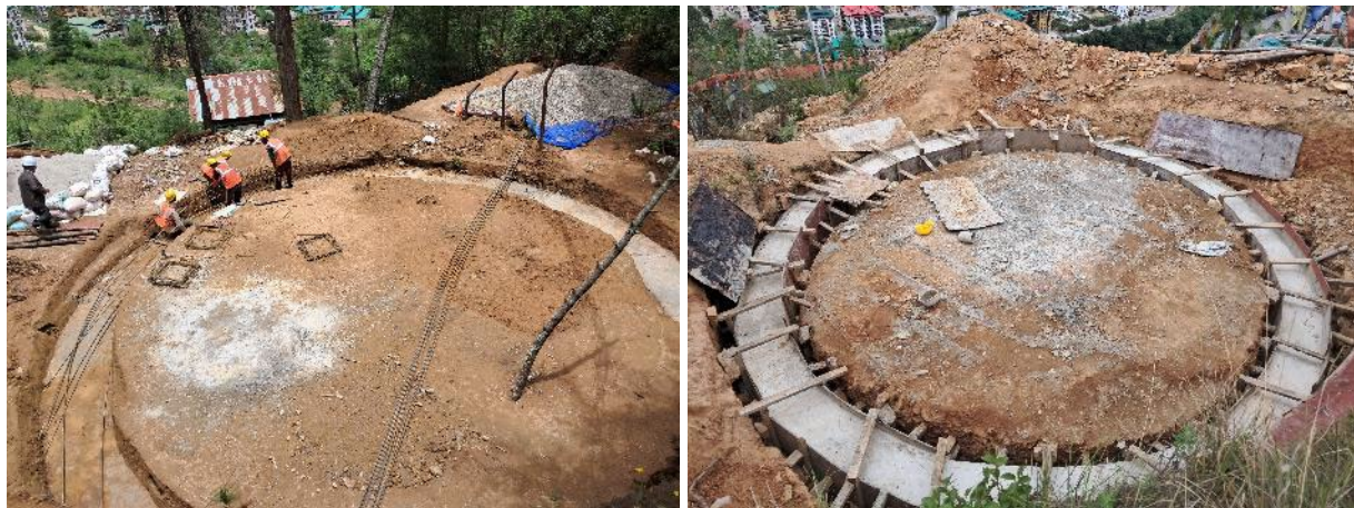
Photo 28 a & b. 230 and 100 cum reservoir tanks
