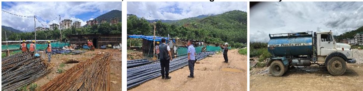
Photo 16 a, b & c. Material storage and machinery
