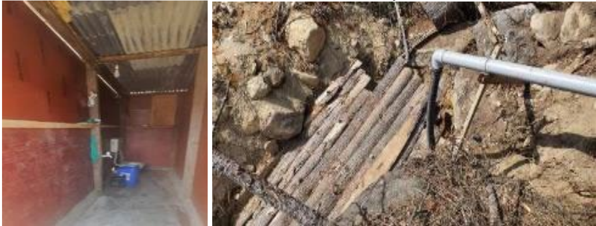
Photo 5 a & b. Staff toilets with septic tank
