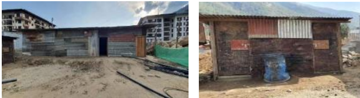
Photo 15 a & b. Site office and toilet
