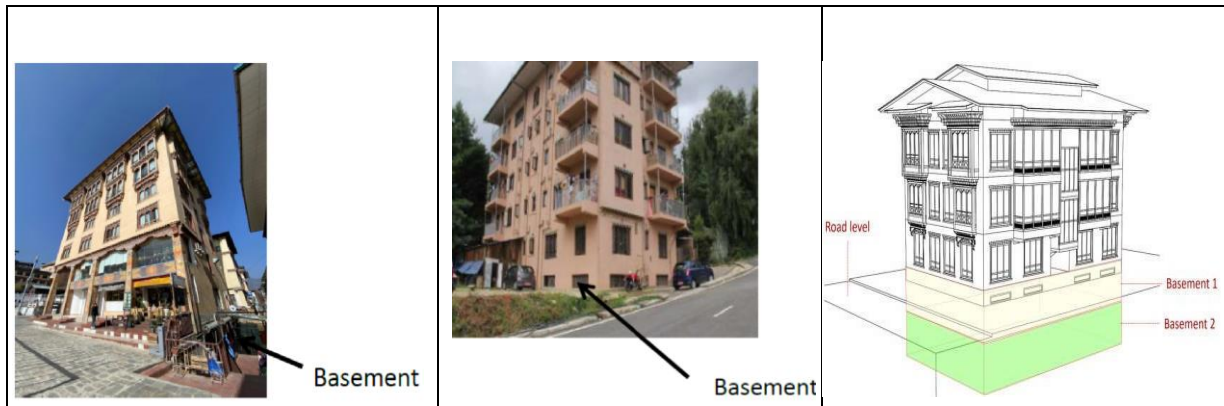
Figure 15: Examples of different types of Basements (Source: DHS and CAS, Thimphu Thromde)
