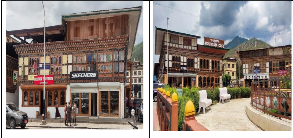
Figure 9: Joint construction on one plot (Eg. In Paro Town)
