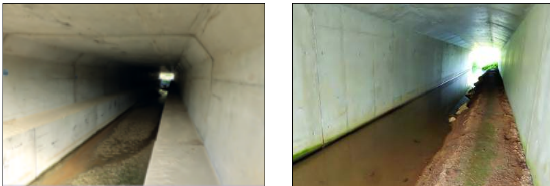
Figure 34: Examples of Modified Culvert Designs Enabling Wildlife Passage
