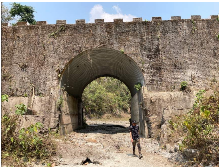
Figure 32: Large Mammal Underpass on Raidak–Lhamoizhingka Road
