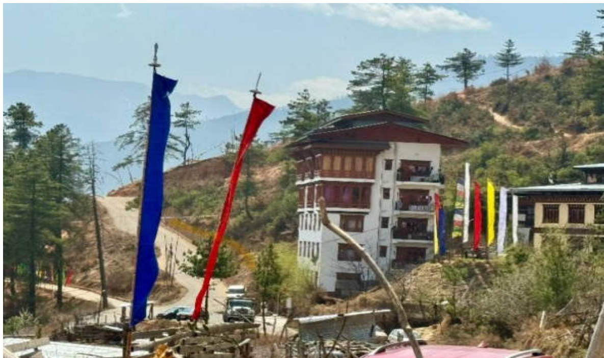
Image 2: Realignment of trunk line pipe section due to possible slope instability below lhakhang steep gradient
