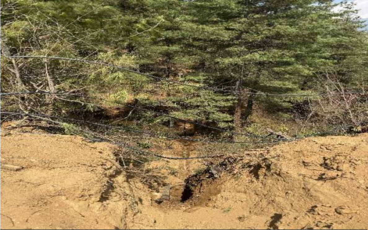
Image 1: Realignment of trunk line pipe section due to steep gradient
